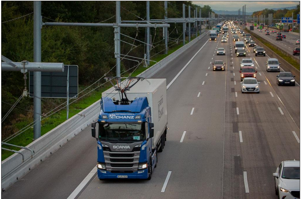
Figure 5.4: Photograph showing the concrete road-side crash barrier installed for the German ERS demonstration project.
